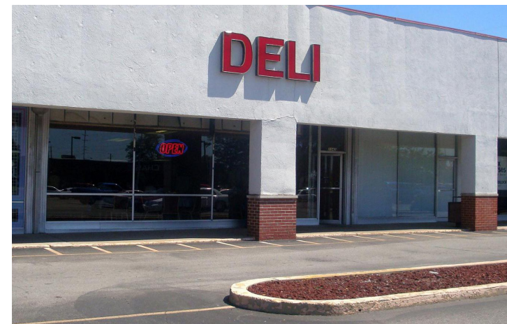
Unacceptable Signage Placement
