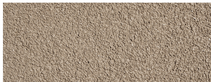
Exterior insulation and finishing system (EIFS)
